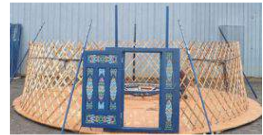
3a. attach bagaans (central posts) to toono (top dome)....
