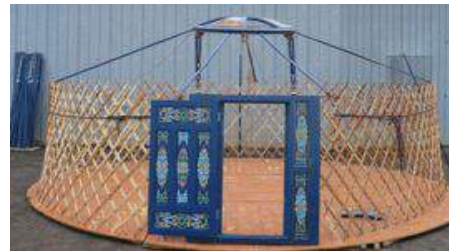
4. put huns (roof rafters). adjust tension with circular tension rope and make sure the toono is placed symetricaly in the circle and towards the door.
