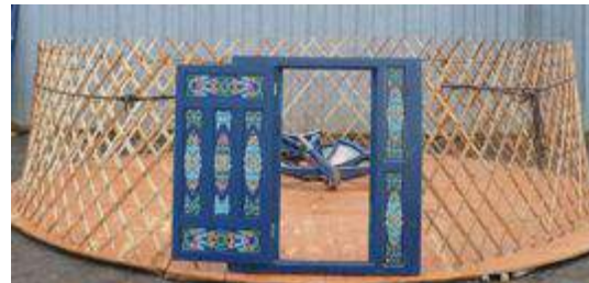
2. connect walls in a circle and add tension rope
