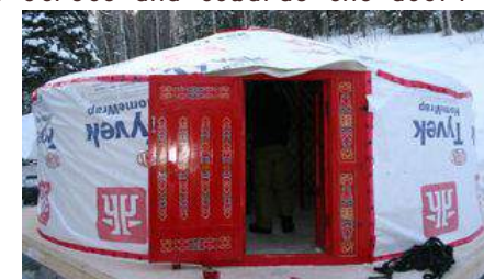
7a. recommended option: add layer of house wrap - prepare toono BEFORE phase 1 !
